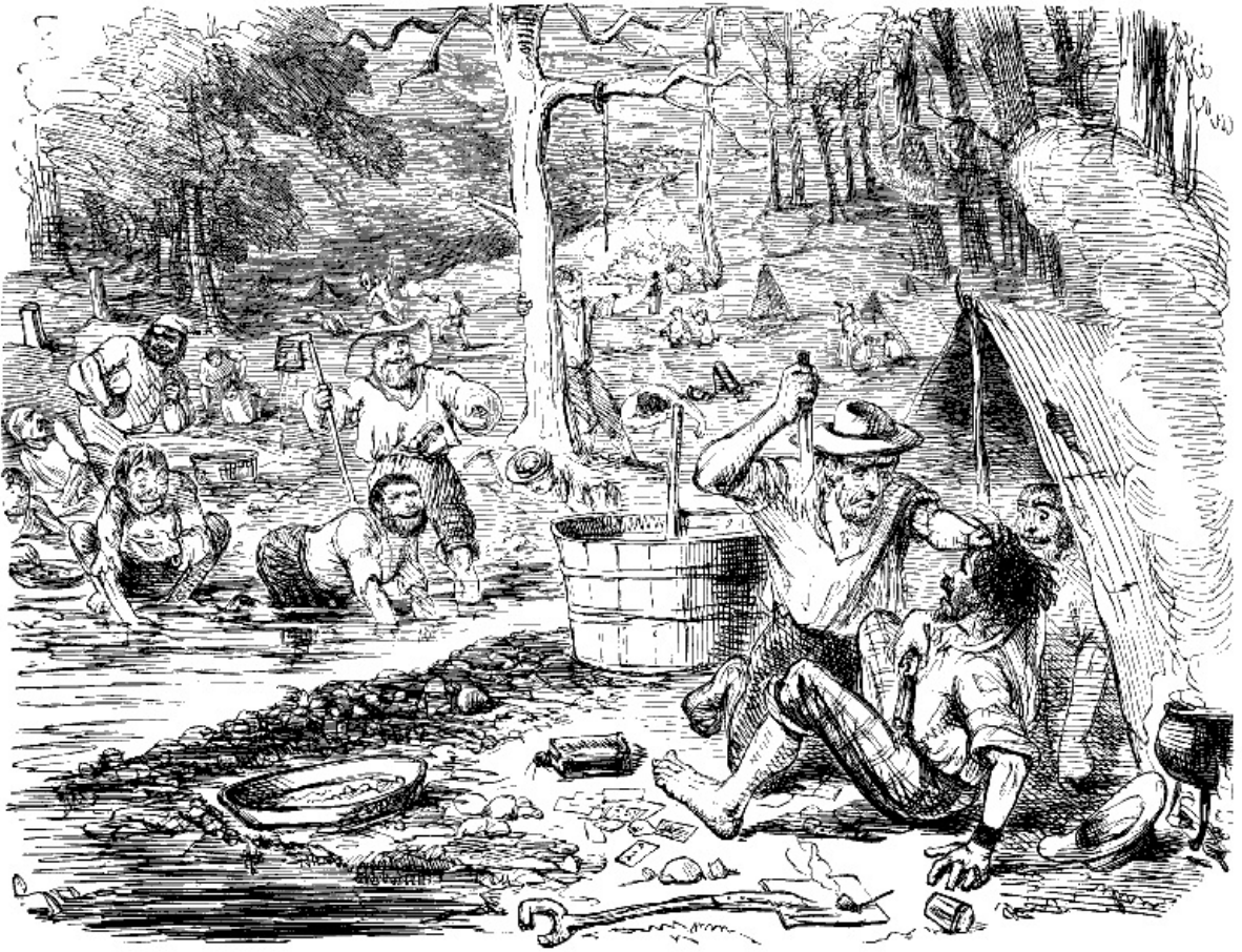
A GOLD FIELD IN THE "DIGGINS."
