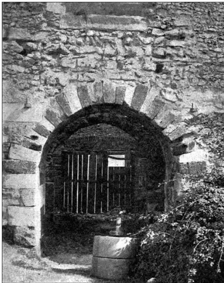
FIG. 16. THE WATER-GATE, PORCHESTER
