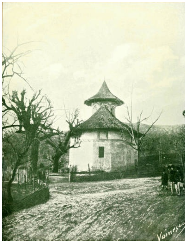
"THE ROOFS ARE ALWAYS OF SHINGLE" (p. 44).
