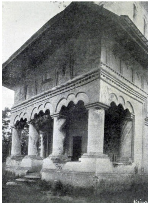
"THEIR PRINCIPAL FEATURE BEING THE STOUT COLUMNS THAT SUPPORT THE PORCH IN FRONT" (p. 44).
