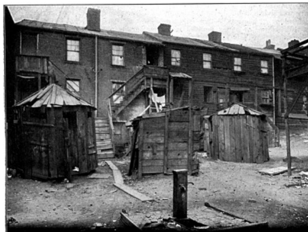
YARD SHOWING BATTERIES OF PRIVY VAULTS AND DILAPIDATED CONDITION OF STEPS LEADING TO THIRD STORY. TWO ROOM APARTMENTS RENT FOR $12 PER MONTH.
