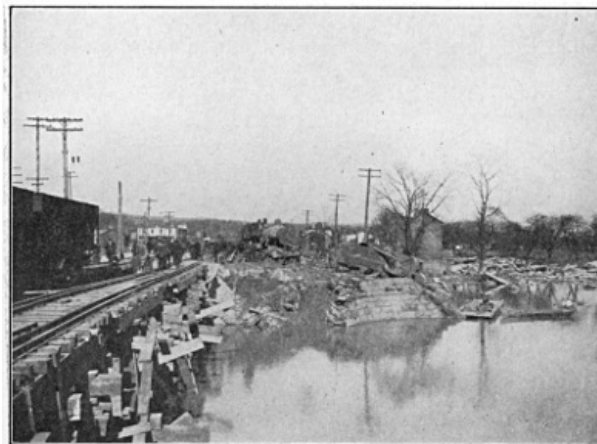
RAILROAD BRIDGE DESTROYED BY FRESHET. THREE MEN WERE KILLED IN THE WRECK WHICH FOLLOWED.
