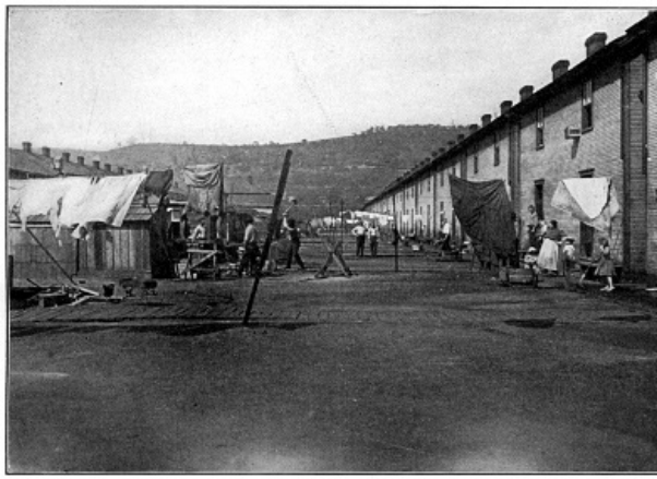
SCHOEN: Box-like rows of company houses with out-buildings between.
