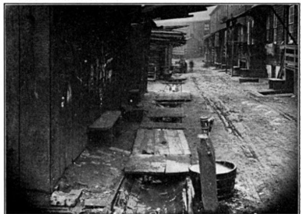
PIPE EMPTYING MILL-WATER INTO OPEN DRAIN BETWEEN ROWS.
