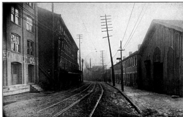
WEST CARSON STREET AT TIME OF FIRST INSPECTION.
