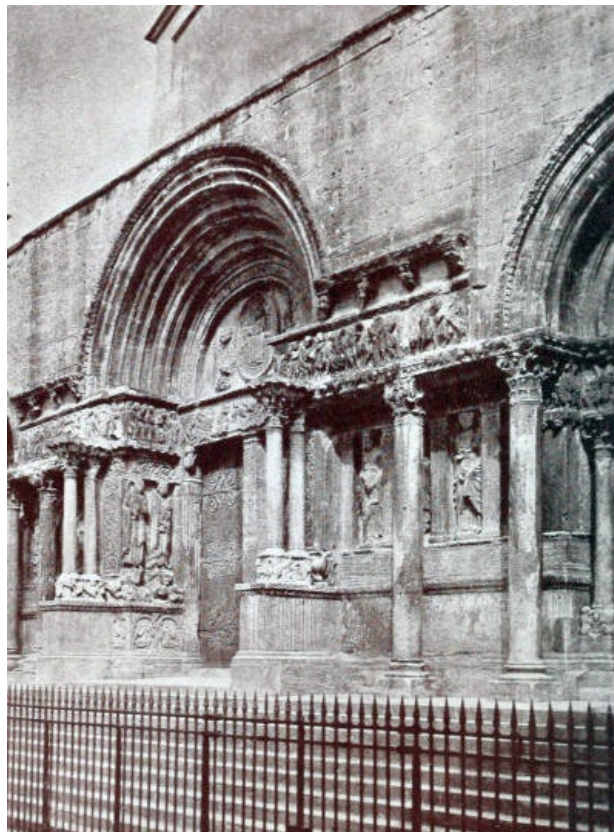
SAINT-GILLES, THE CENTRAL PORCH
