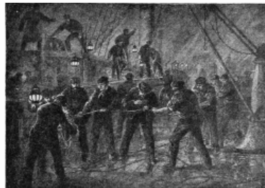
FIG. 39.—“Foul in Tank” while Paying out.
