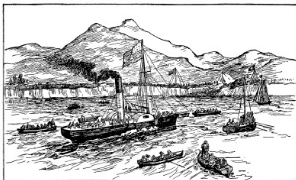
FIG. 14.—Landing the Irish End of the Cable.
