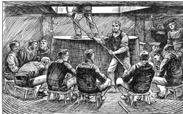
FIG. 13.—Coiling the Cable on Board.
