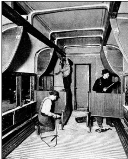
Interior work. The steel framework for seats and berths
