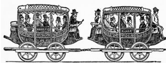
Early passenger cars, designed after the then prevalent type of horse coach. These cars were part of the train that ran on the formal opening of the Mohawk & Hudson Railroad (the first link of the New York Central System) on July 5, 1831.
