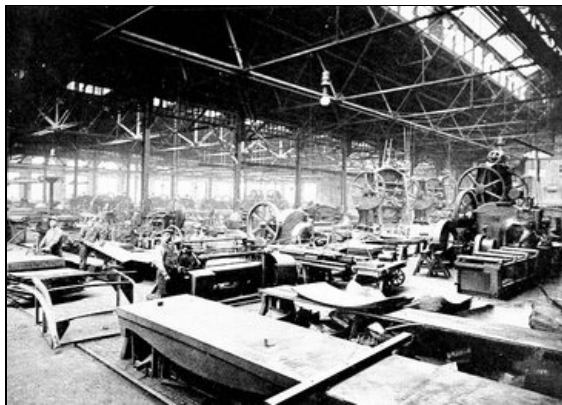
View of machine section. Steel Erecting Shops
