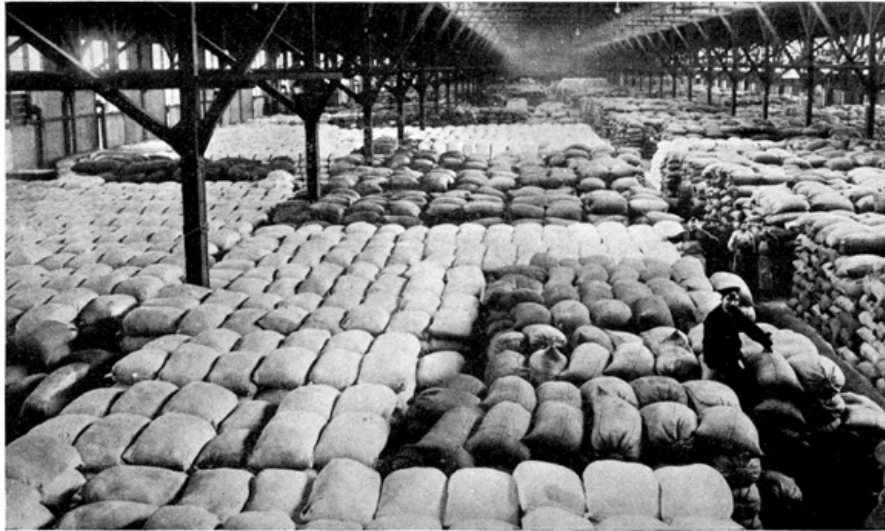
View of a Grain Storage at Hamburg.
