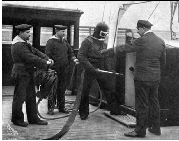
Hose from bellows supplies fresh air to man with smoke helmet.
