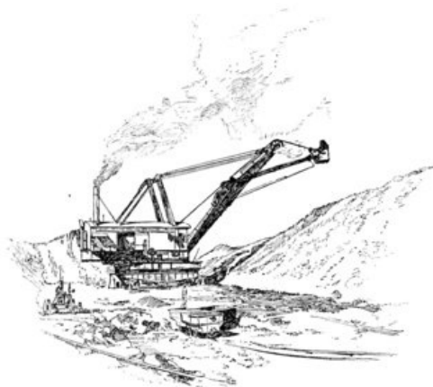
THE STEAM SHOVEL SHOVELS BY MEANS OF A WIRE ROPE
