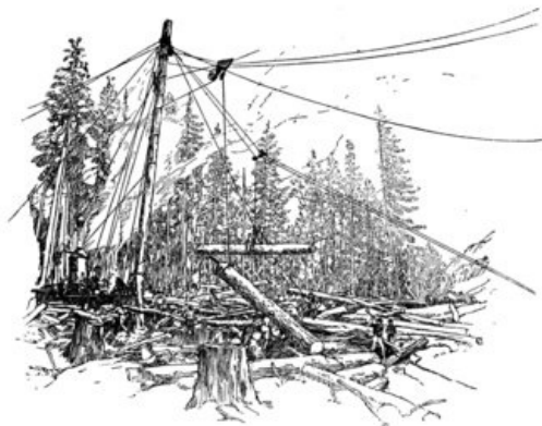
LOGGING—HANDLING BIG FELLOWS WITH WIRE ROPE
