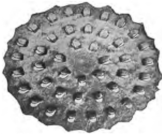
FIG. 30.—Detail of Perforated Plate A.
