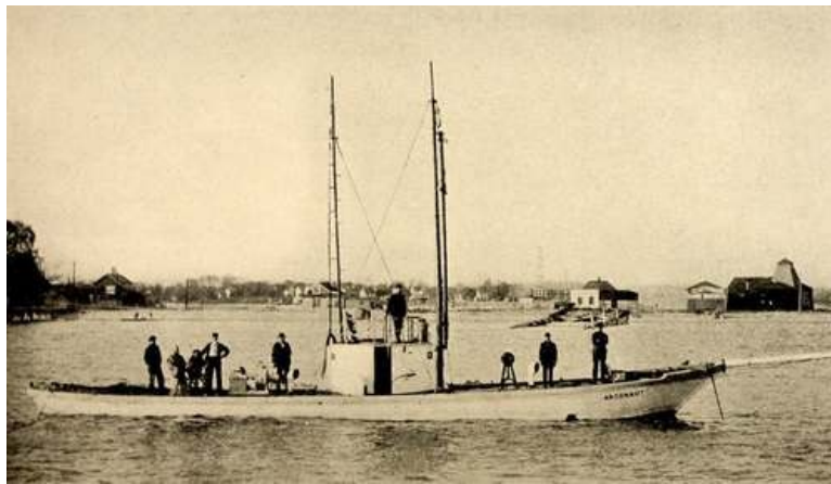
THE "ARGONAUT," AFTER BEING LENGTHENED AND REBUILT, IN 1898, SHOWING SHIP-SHAPED, WATERTIGHT, BUOYANT SUPERSTRUCTURE
