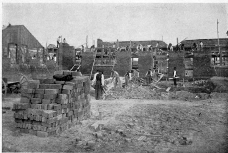
STUDENTS AT WORK ON NEW TRADES-SCHOOL BUILDING.
