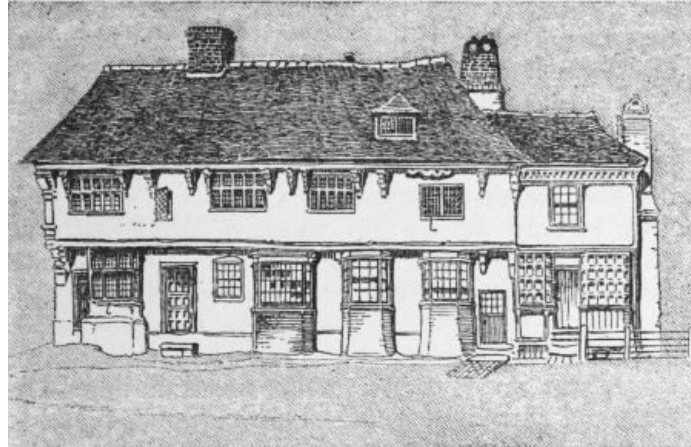
OLD HOUSES AT ELHAM.
