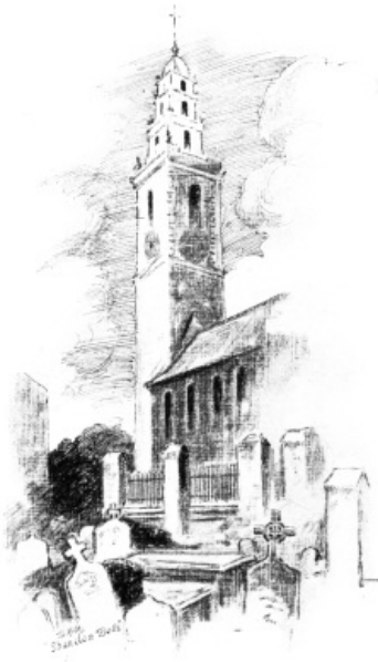
SHANDON CHURCH TOWER.
