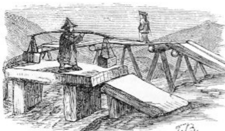
CHINESE SLAB AND TRESTLE BRIDGE.
