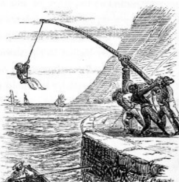
LANDING BY SWINGING DERRICK.
