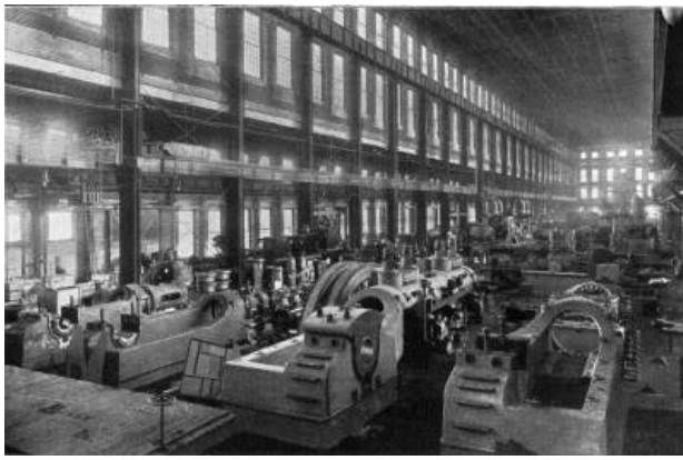
SOUTH END OF ERECTING SHOP, WEST ALLIS WORKS Allis-Chalmers Company, Milwaukee, Wis.
