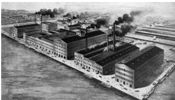
BROOKLYN, N. Y., PLANT OF THE H. W. JOHNS-MANVILLE CO.
