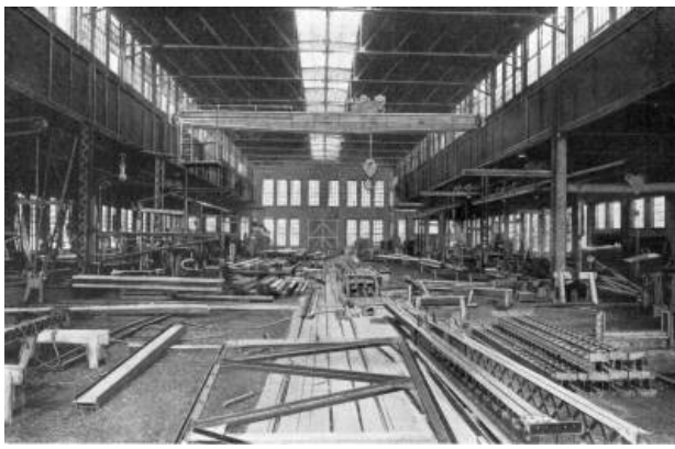
A VIEW IN THE STRUCTURAL SHOP OF THE MINNEAPOLIS STEEL & MACHINERY CO., MINNEAPOLIS, MINN.
