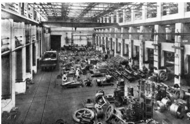
AIR-COMPRESSOR ERECTING ROOM, CLAREMONT, N. H., FACTORY, SULLIVAN MACHINERY CO.
