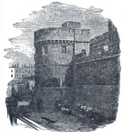
THE FLINT TOWER.
