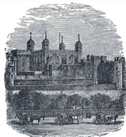
GENERAL VIEW OF THE TOWER.
