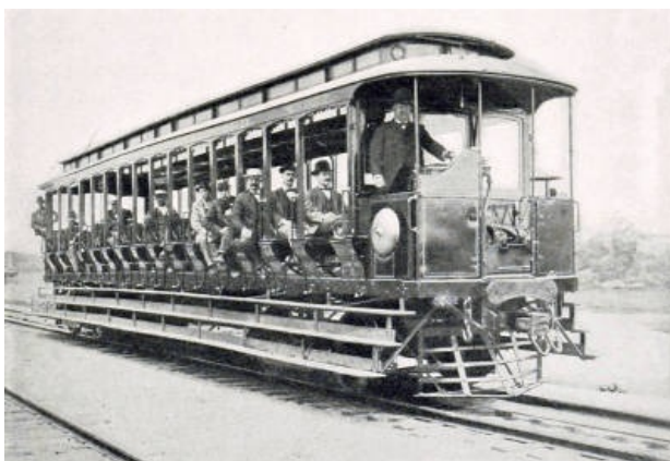
FIG. 30.—VIEW OF A SECTION OF THE NEW YORK, NEW HAVEN AND HARTFORD RAILROAD, EQUIPPED WITH THE THIRD-RAIL SYSTEM.
