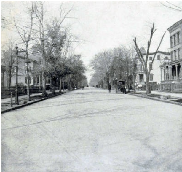
ASPHALT PAVEMENT ON CLINTON AVENUE, BROOKLYN.
