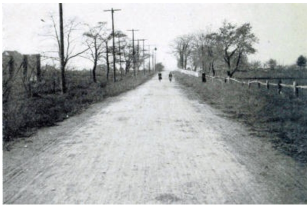
KING'S HIGHWAY, BROOKLYN; SIXTEEN FEET IN CENTER OF ROAD MACADAMIZED.
