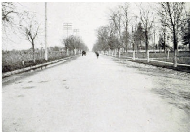
EIGHTEENTH AVENUE, BROOKLYN; MACADAMIZED FULL WIDTH OF ROADWAY AND GUTTERS PAVED, WITH NO PROVISION FOR SURFACE DRAINAGE.
