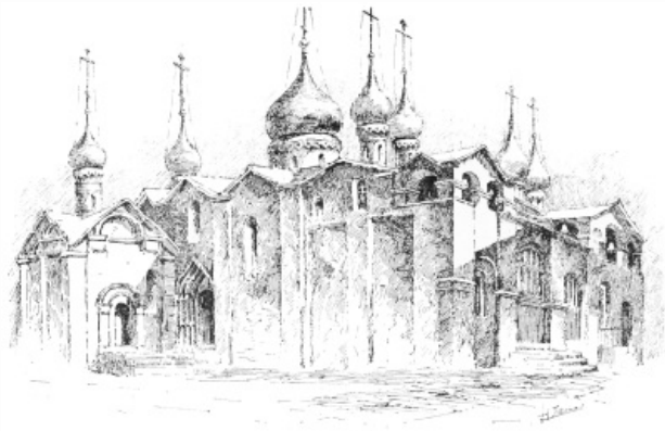
SPASS NA BORU (ST SAVIOUR'S IN THE WOOD)
