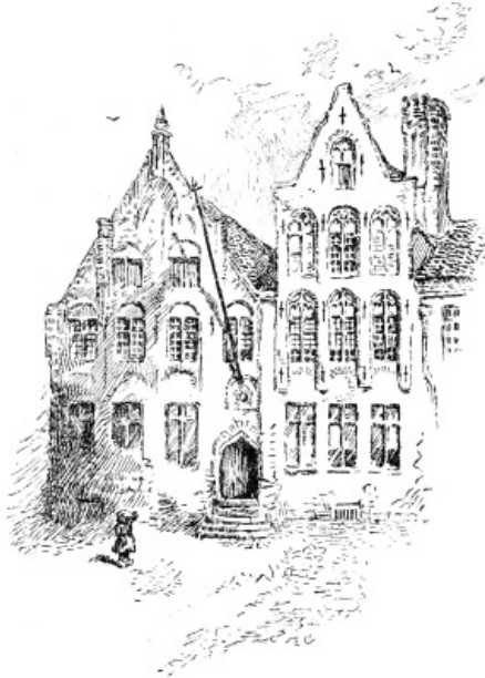
OLD HOUSES AT DAMME
