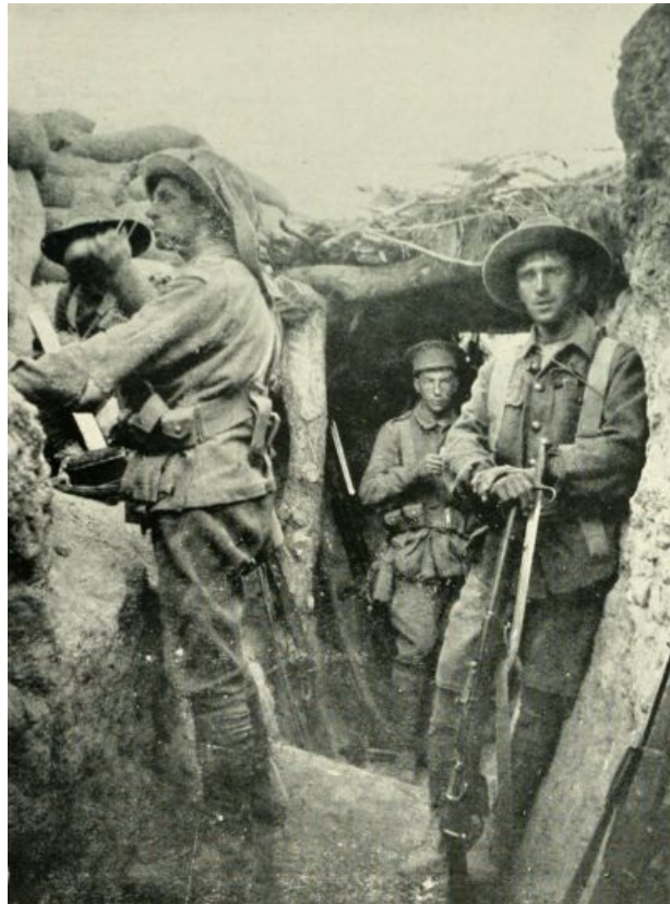
THE OVERHEAD COVER OF PINE LOGS IN THE CAPTURED LONE PINE TRENCHES.
