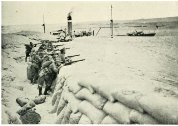
AUSTRALIANS MANNING A COMMUNICATION TRENCH LEADING TO ISMAILIA FERRY POST.
