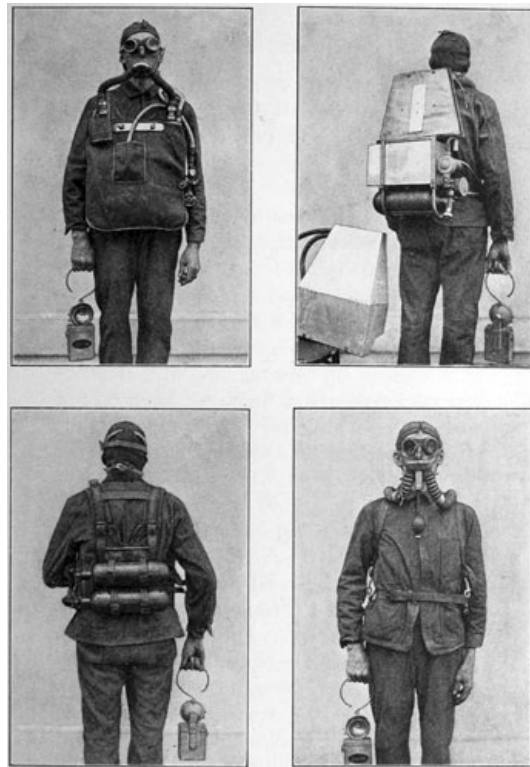
Breathing-apparatus necessary in going into "gassy" galleries.
