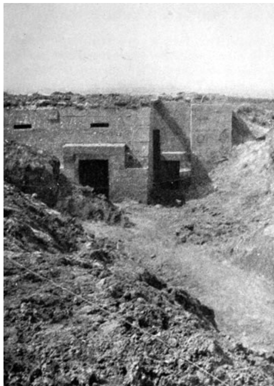
View from rear of a typical German reinforced concrete machine-gun emplacement. Taken on the Hindenburg line south of Arras.
