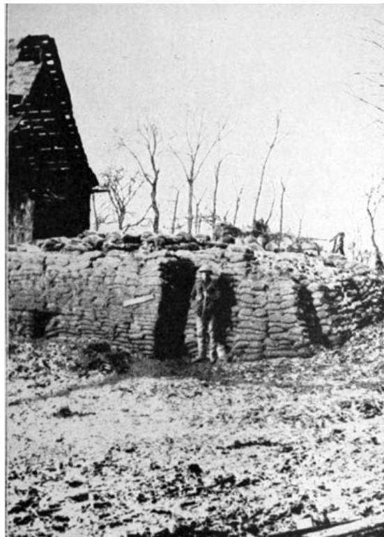
A cellar, protected by sand-bags, in the village of Hébuterne, used as a shelter by engineer officers.
