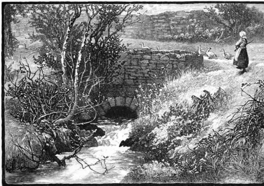
THE FIRST BRIDGE OVER THE THAMES.
