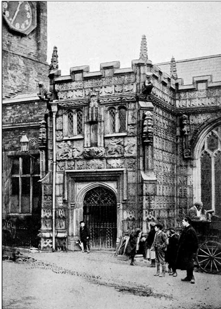
LAUNCESTON CHURCH PORCH
