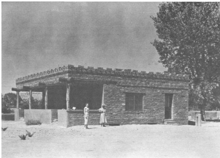
The Earl Morris house about 1933; today the Aztec Ruins Visitor Center.
