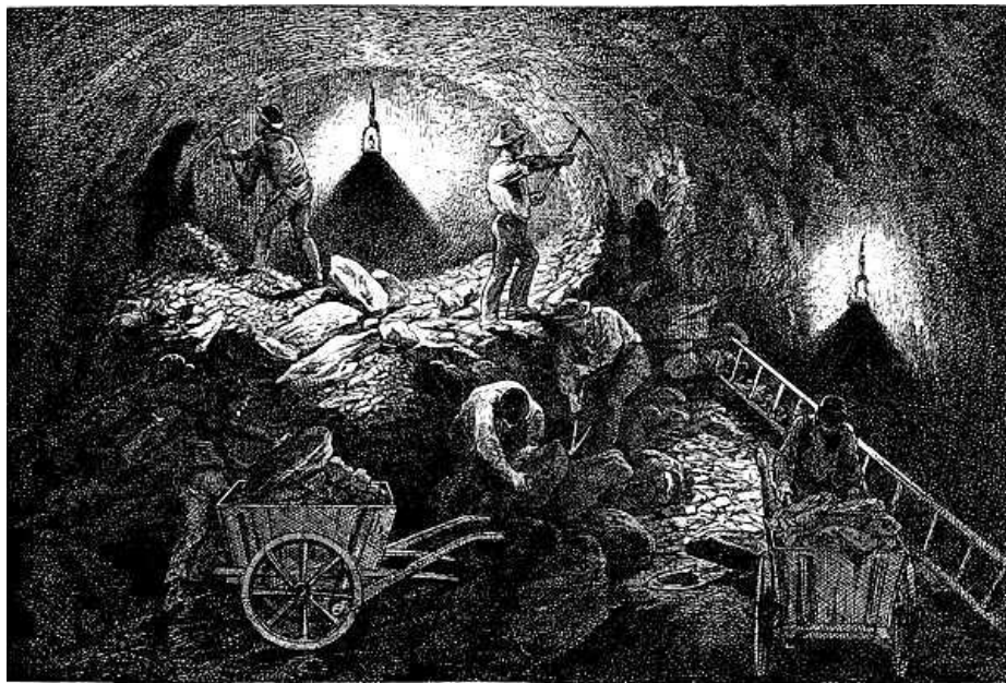
THE EXCAVATION OF DEUTZ AND GELDERMANN'S NEW CELLARS AT AY.
