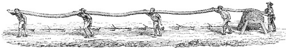
UNROLLING MATTING FOR ROOFING THE VINES WITH.
