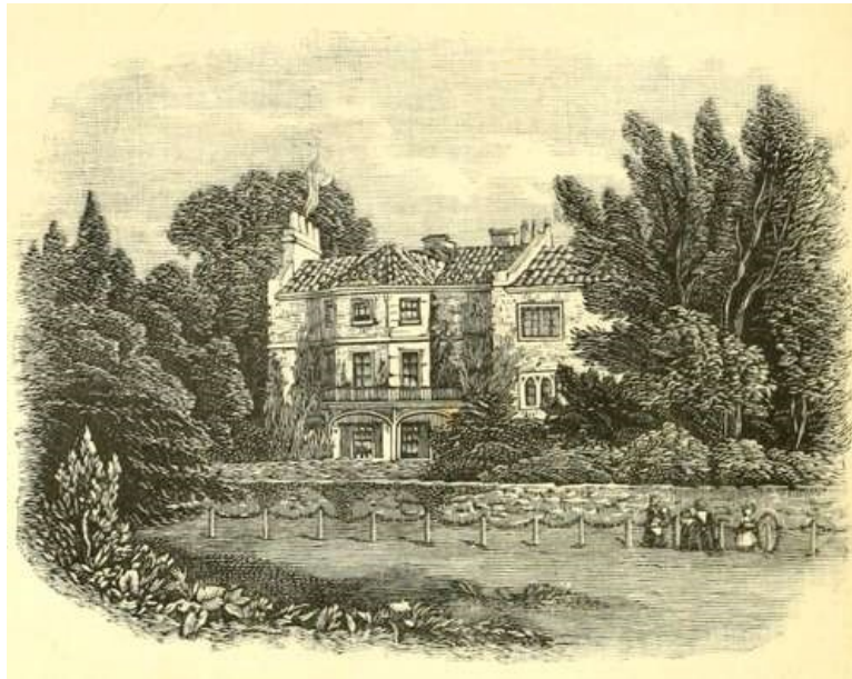
KITTY CLIVE'S HOUSE, TWICKENHAM.
