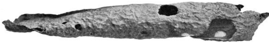
COPPER DRIP PIPE AFTER SEVENTEEN DAYS' EXPOSURE IN SALT WATER TO THE ACTION OF ELECTRICITY. Half size.
