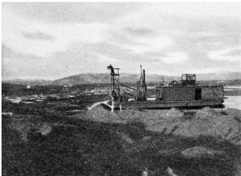
ERECTING A STEAM PUMP (NOME).
