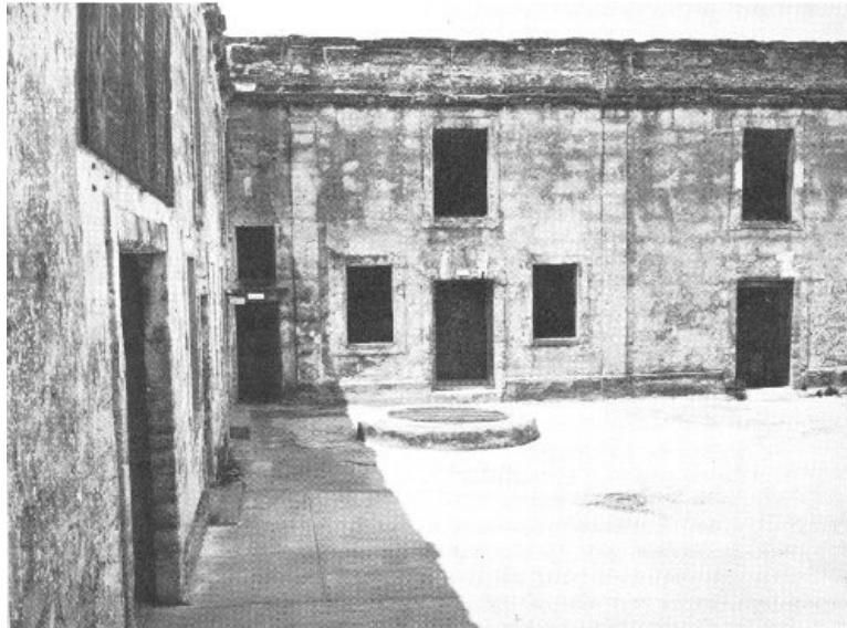
MOST OF THE ROOMS OPEN INTO THE SQUARE COURTYARD OR PARADE OF THE FORT. THE WELL IN THIS CORNER FURNISHED THE ONLY PALATABLE WATER SUPPLY FOR REFUGEES INSIDE THE FORT DURING TIMES OF SIEGE.
