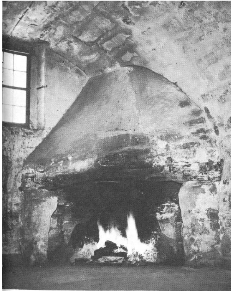
THE LARGE CORNER FIREPLACES IN THE GUARDROOMS WERE USED BOTH FOR HEATING AND COOKING.
