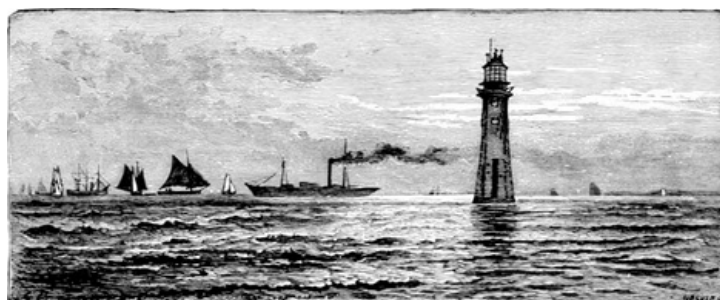
THE PERCH ROCK LIGHTHOUSE.
