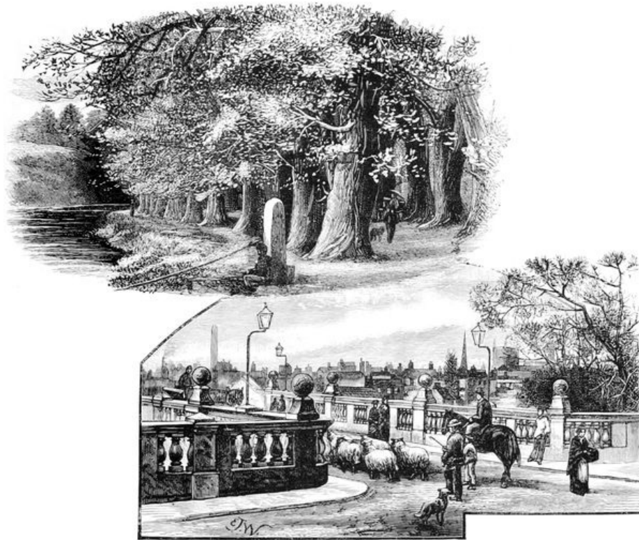
ENGLISH BRIDGE, SHREWSBURY ( p. 91 ).
