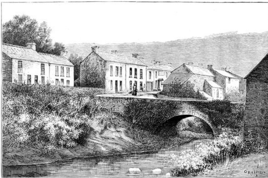
OUTSKIRTS OF NEATH.
