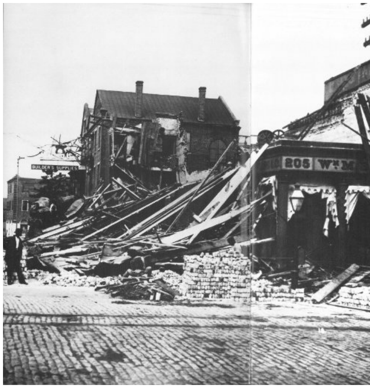
Many buildings in Charleston, South Carolina, were damaged or destroyed by the large earthquake that occurred August 31, 1886.
