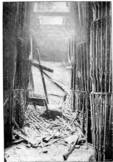
FIG. 24.—EXPLOSION AT TOWER OF LONDON—THE BANQUETING HALL.
