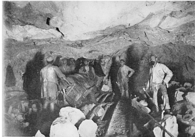
DRIVING AN "END" IN MAY CONSOLIDATED MINE, JOHANNESBURG
