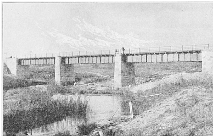
MACHECKIE RAILWAY BRIDGE ON THE SALISBURY LINE, MASHONALAND RAILWAY
