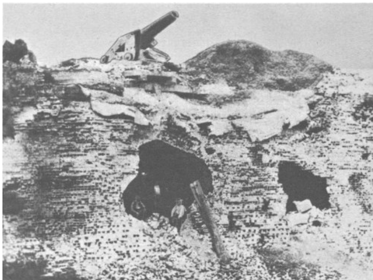
"No works of stone or brick can resist the impact of rifled artillery of heavy calibre." From The Photographic History of the Civil War.
