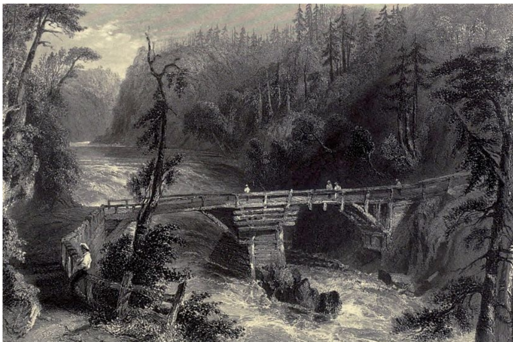
Bridge near Quebec.
