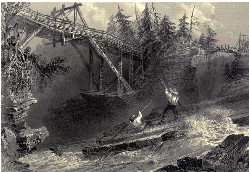
Timber Slide and Bridge on the Ottawa.
