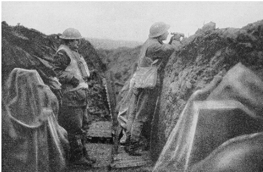
A First Improvement in Trenches: A Dry Trench in the Front Line.
