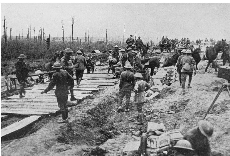
Australian Pioneers construct a Roadway while the Battle is proceeding.
