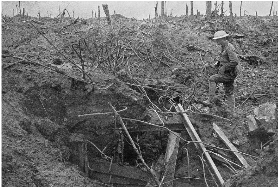
The Effect of a 9.2 British Shell on a Reinforced Concrete German Dug-out. The dug-out was some feet below the surface of the ground and the concrete roof and wall were over 2 feet thick.
