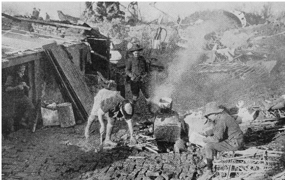
A Cook-house in Montauban.
