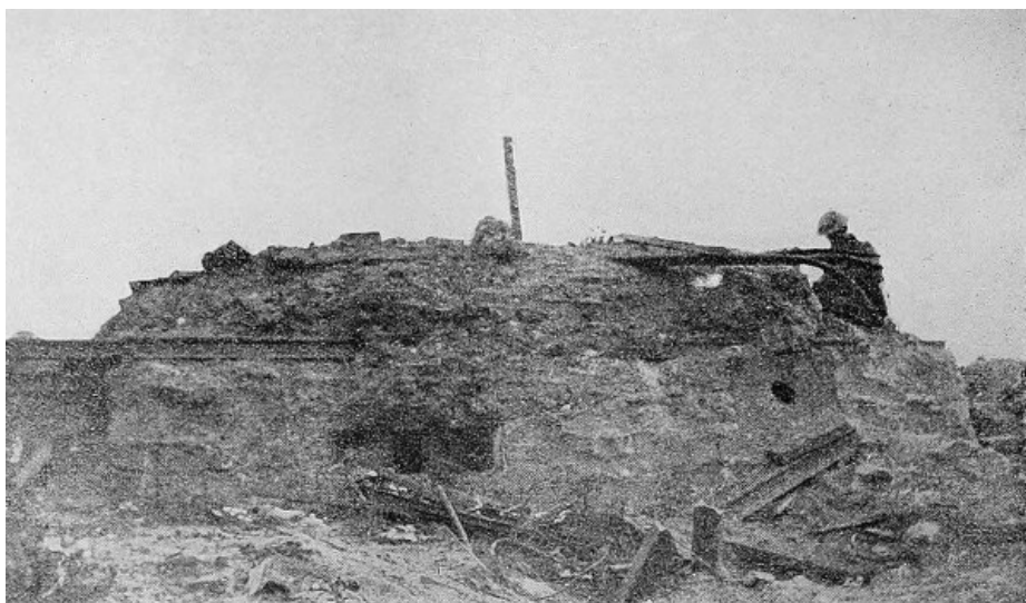
A German Concrete and Steel Blockhouse of the type which Australians first met at Messines.
