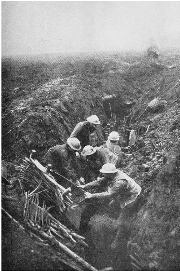
Engineers beginning on the Track across "The Maze," part of the old German Front Line which had been held all the Winter.
