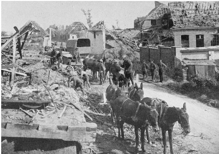
Clearing the Roadway.
