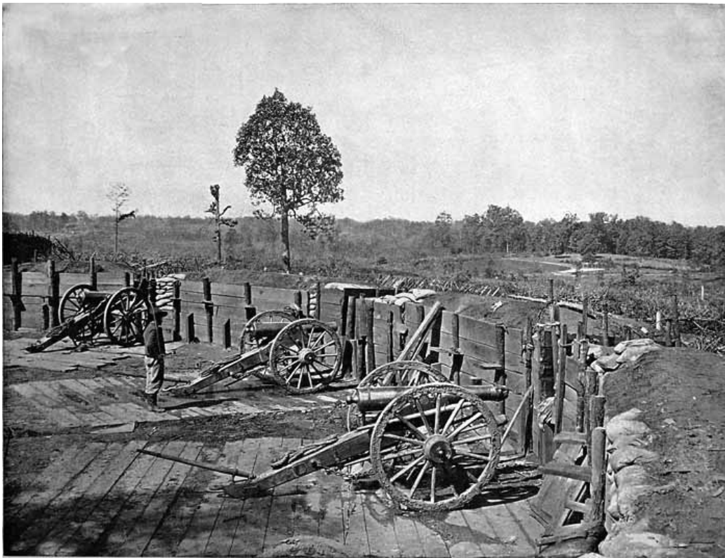
INTERIOR OF CONFEDERATE FORTIFICATION.
