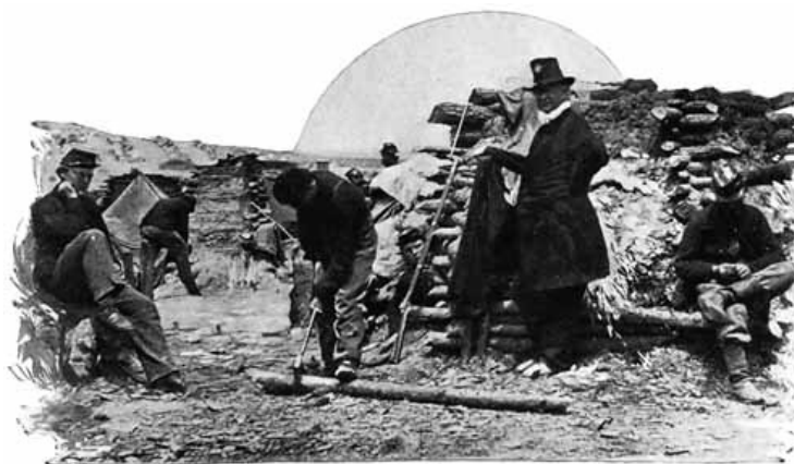
CONSTRUCTING WINTER QUARTERS.
