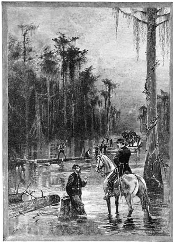
CONSTRUCTING MILITARY ROAD THROUGH SWAMP.
