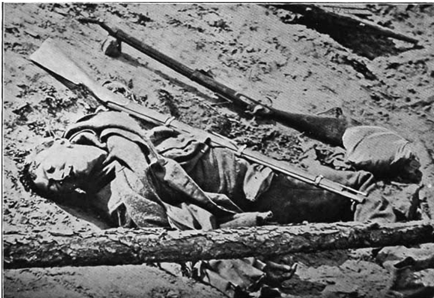
A DEAD CONFEDERATE IN THE TRENCHES.
