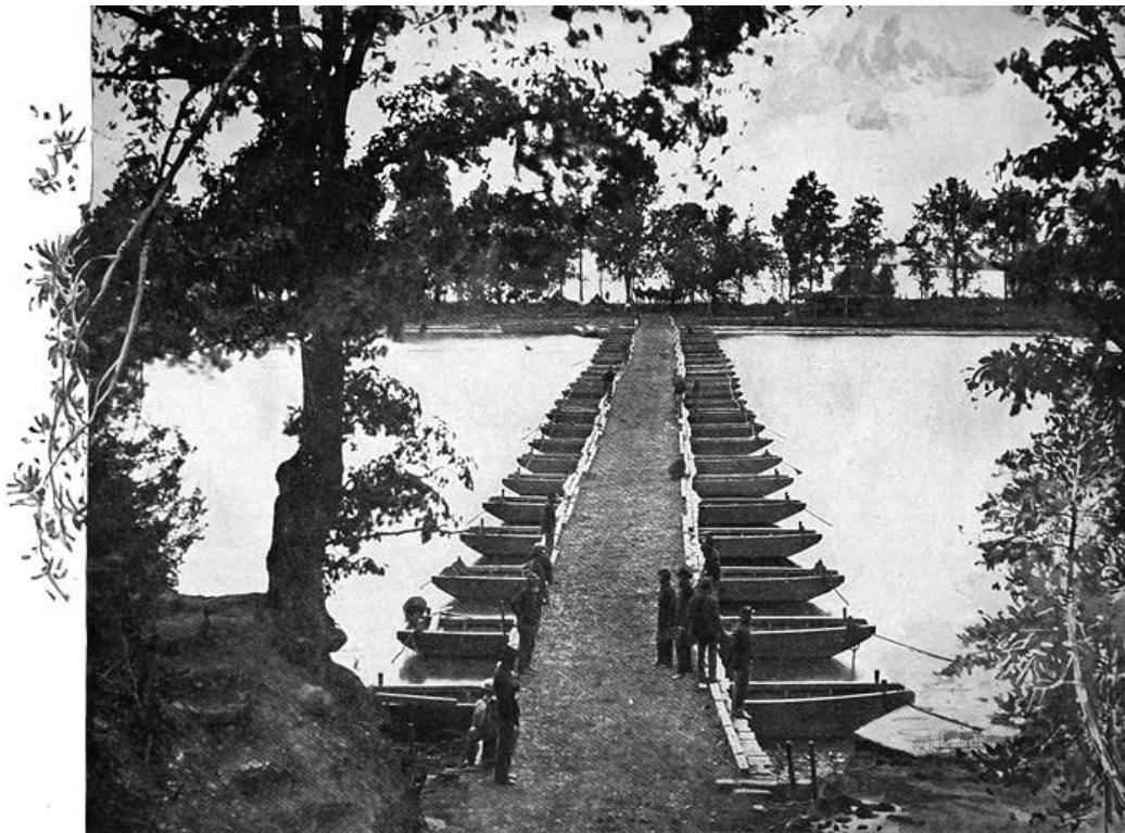
PONTOON BRIDGE AT DEEP BOTTOM ON THE JAMES RIVER.
