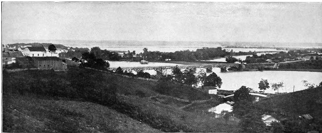
AQUEDUCT BRIDGE, POTOMAC RIVER.
