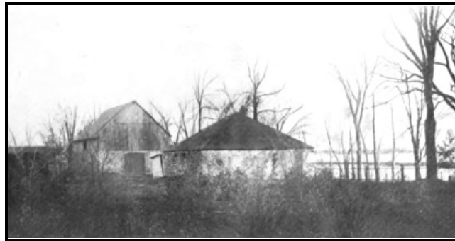
KING'S FORT AND POWDER HOUSE (AS STANDING TODAY) FORT CALLERIER
