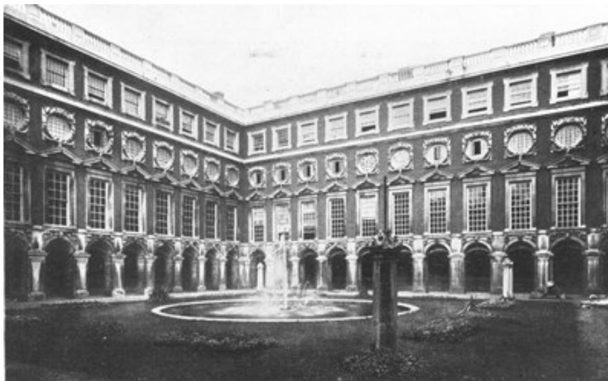
FOUNTAIN COURT HAMPTON COURT PALACE
