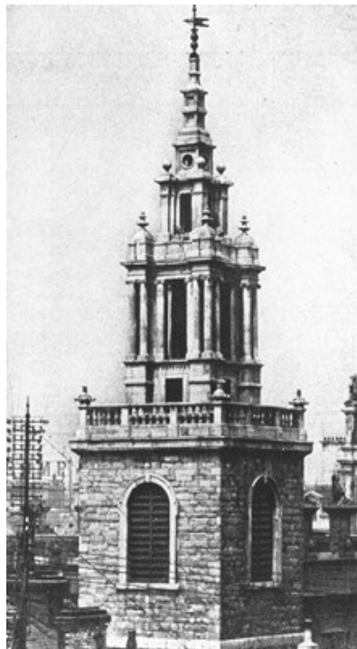
STEEPLE, ST. STEPHEN'S WALBROOK LONDON
