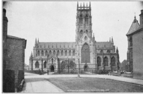
CHURCH OF ST. GEORGE, DONCASTER, YORKS, ENGLAND, EXTERIOR.
