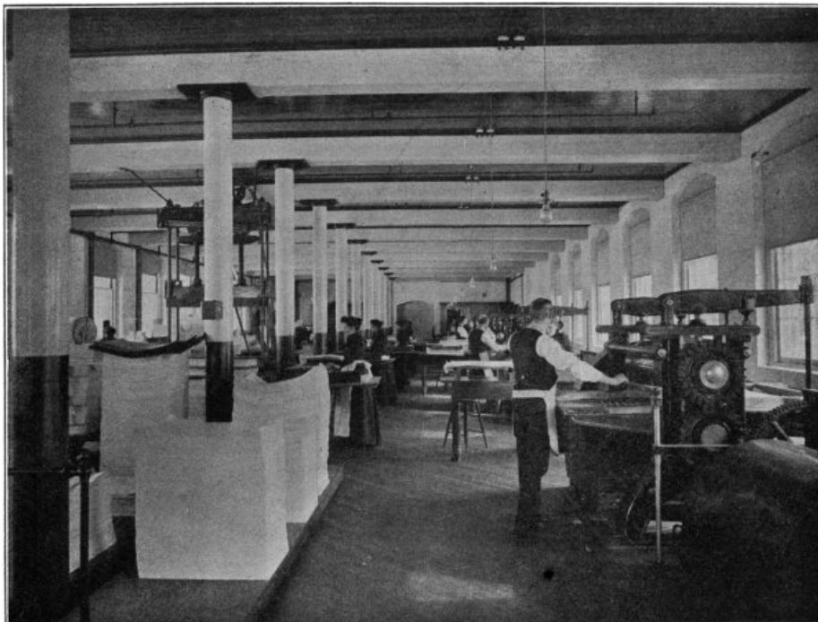
FINISHING-ROOM, CRANE & CO. The machine on the right is a plater.
