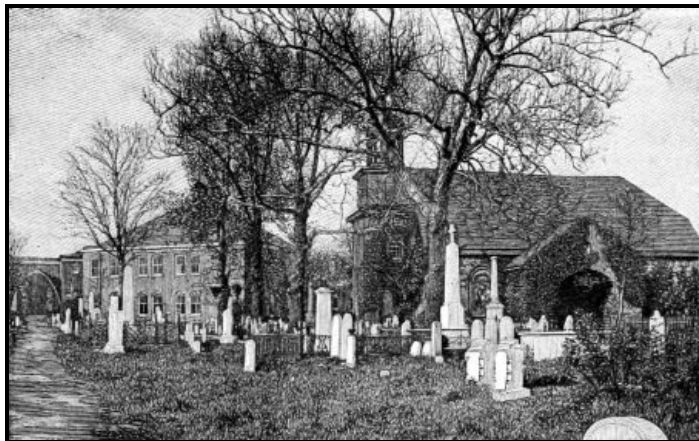
Old Swedish Church at Wilmington, Delaware.
