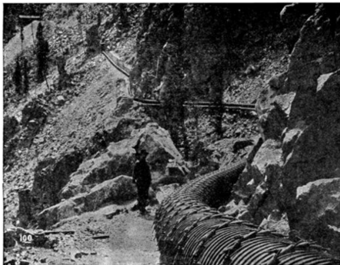
FIG. 20.—Wood Pipe Line to Pike's Peak Power-house.
