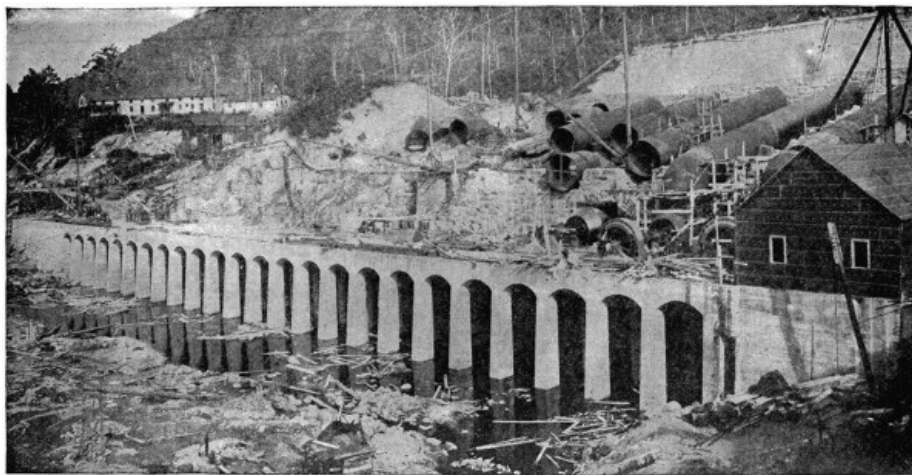
FIG. 32.—Foundation of Power-station at Spier Falls.
