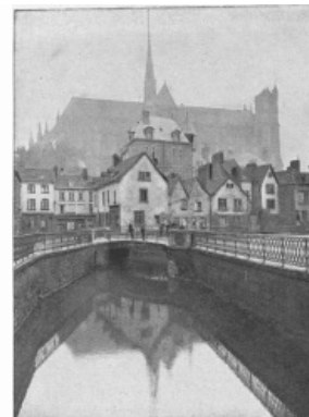
OLD BISHOPS' PALACE (in front of Cathedral). To the right, RUE DU DON.
