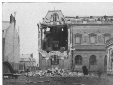
MUSEUM: RIGHT WING OF REAR FAÇADE DAMAGED BY AERIAL TORPEDO IN 1918.
