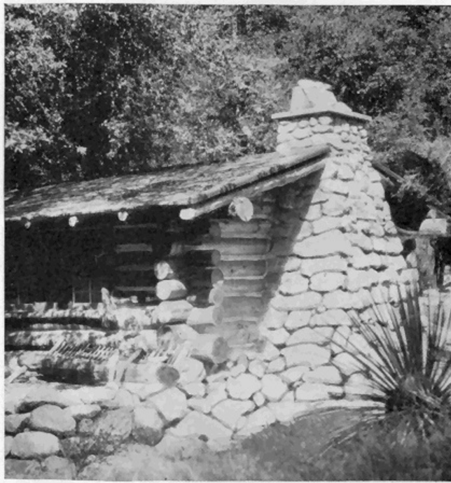
FIGURE 4.—Short chimneys are frequently provided for low bungalows, for architectural reasons. This flue is ample in size but not high enough for use with a stove. The stone masonry has been laid to harmonize with the rustic surroundings.
