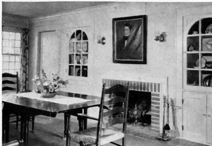
FIGURE 31.—This 36-inch-wide fireplace does not seem too large for the small room, but its size would have been accentuated by the use of a mantel.
