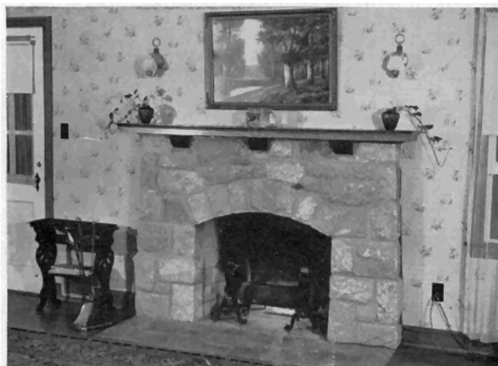
FIGURE 38.—This well-designed small stone fireplace was built in accordance with the principles given in this bulletin. It is a good heater and does not smoke. The jambs are wide enough to resist the thrust of the arch.
