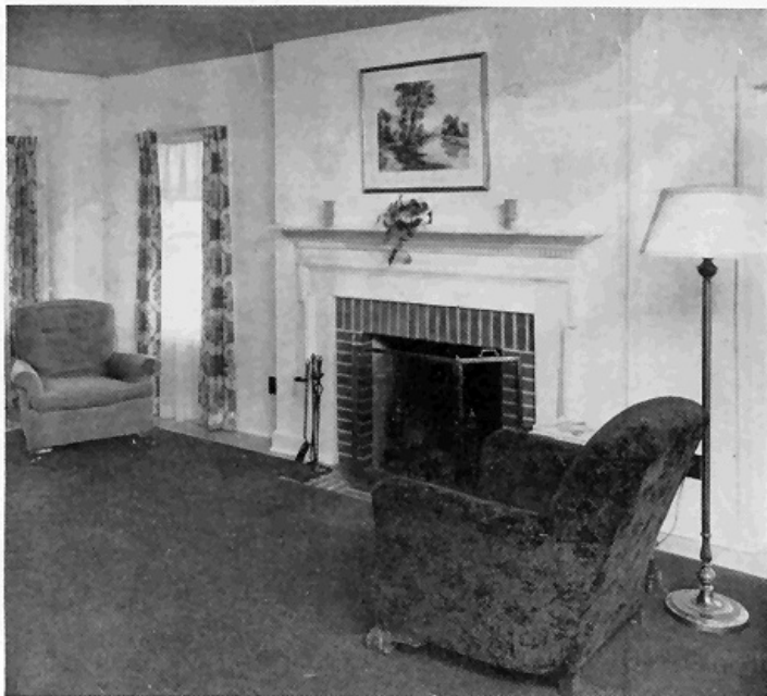
FIGURE 23.—A well-designed commercial mantel that suits the room. Since it is painted the same color as the walls, it does not focus attention, as the handsomely carved formal mantel or mahogany shown in figure 37 is intended to do.
