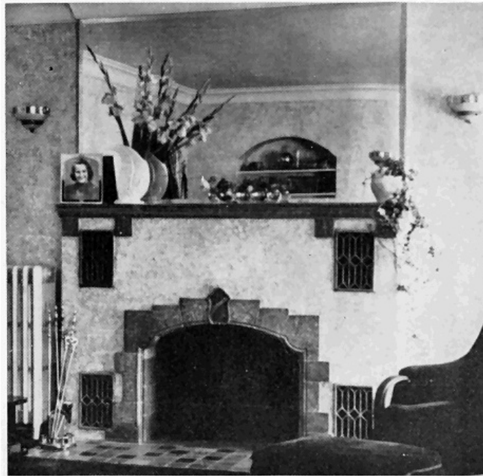
FIGURE 22.—Except for the registers and metallic sides and back, the appearance of modified fireplaces is like that of ordinary ones. An interesting effect is secured by the mirror—the reflection of the opposite wall appears like a recess over the mantel.
