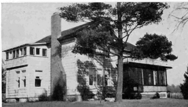
FIGURE 1.—A properly designed and well-built chimney that provides ample draft and protection against fire.
