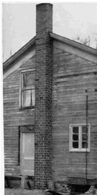
FIGURE 3.—This tall chimney produced good draft for the kitchen range, but the flue was too small for a furnace. When the house was remodeled, its appearance was greatly improved by building the chimney inside.
