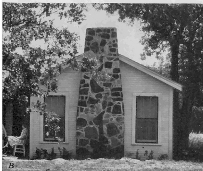
FIGURE 5.—Two pleasingly designed fireplace chimneys that fit into their surroundings. A , This chimney stands in the clear and should provide a good draft; B , a chimney under overhanging
