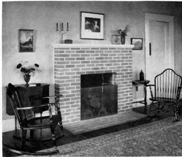
FIGURE 27.—This inexpensive fireplace 32 inches square shows how a plain brick front can be used in a small room.
