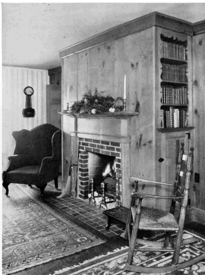
FIGURE 24.—Another good design is this revival of early New England architecture, which is frequently used for remodeling public dining rooms. The random-width pine planks were selected especially for variety in the pattern of the knots. Note the use of otherwise wasted space for bookshelves and closet.
