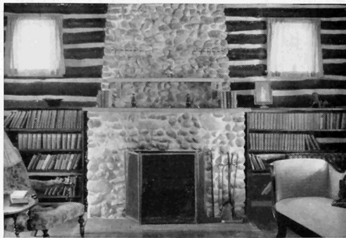
FIGURE 30.—Screens are almost essential to protect the upholstery of nearby furniture from sparks. This fireplace shows artistic use of small stones and makes a pleasing contrast with the log walls.
