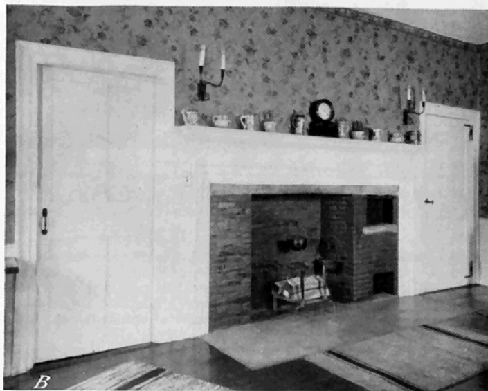
FIGURE 25.— A , A fireplace at Mount Vernon, Washington's home, typical of those used before cooking stoves were introduced. This type of fireplace, if not too large, is often retained ( B ) when a kitchen is remodeled into a living room. Note the Dutch oven at the right, formerly used for baking.
