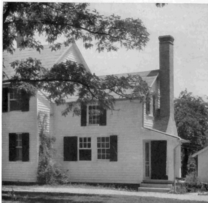
FIGURE 17.—A house in southern Maryland in which the space between the chimney and the house wall shows clearly. The practice of building the chimney in this way is common in the tidewater section of the South.
