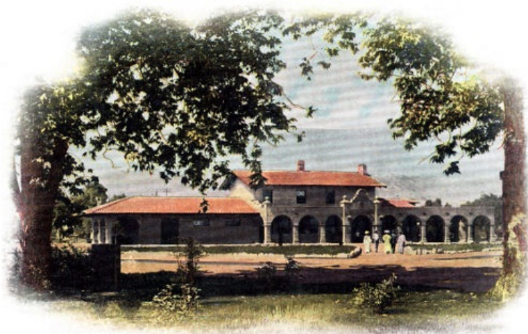
THE SOUTHERN PACIFIC RAILROAD STATION AT SANTA
