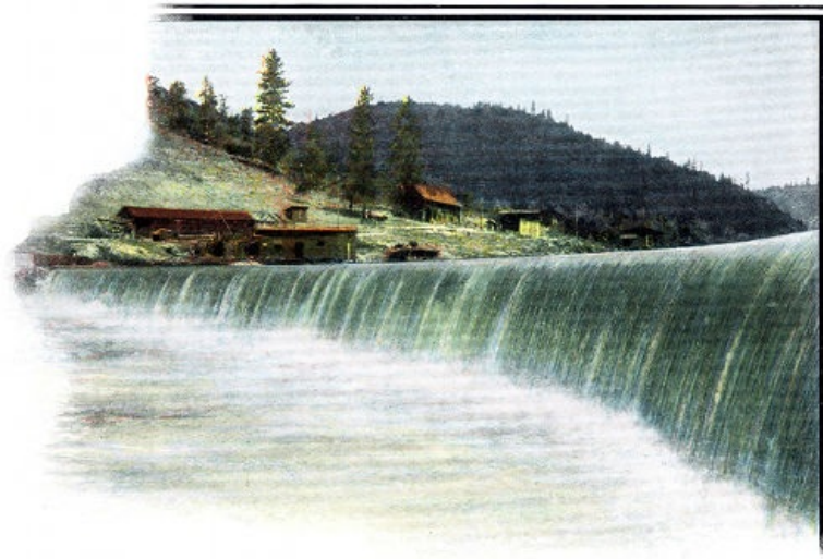
HERE THE CONDOR POWER COMPANY HAS HARNESSSED THE SWIFT FLOWING ROGUE
