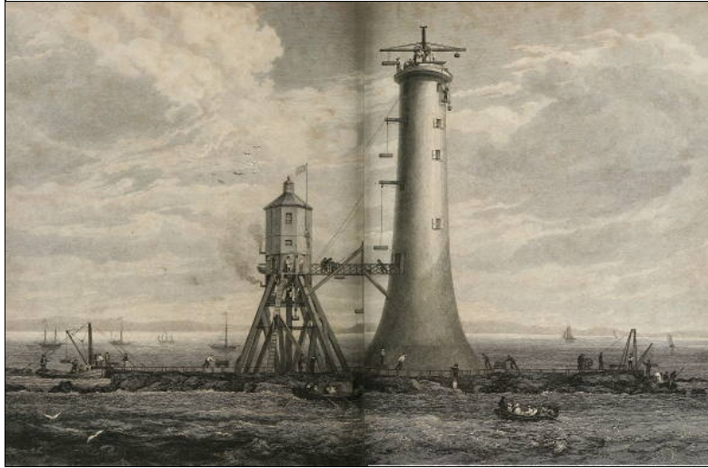
GENERAL VIEW OF THE BELL ROCK WORKS.
